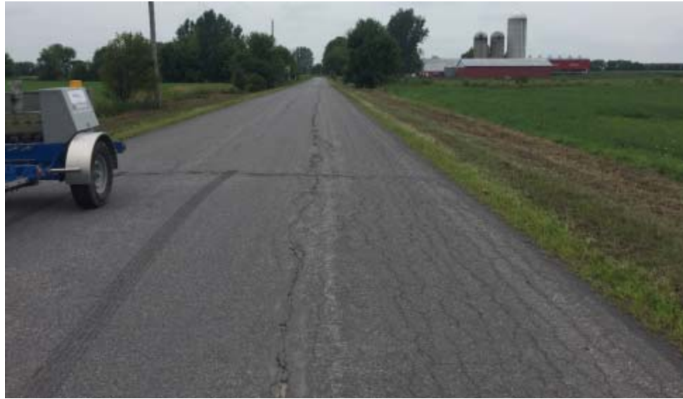
Figure 3-3: Paved Segment of Goldfield Road North (Engtec, 2018)
