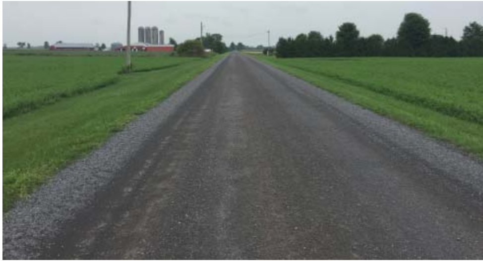
Figure 3-1: Concession Road 6-7; gravel road (Engtec 2018).
