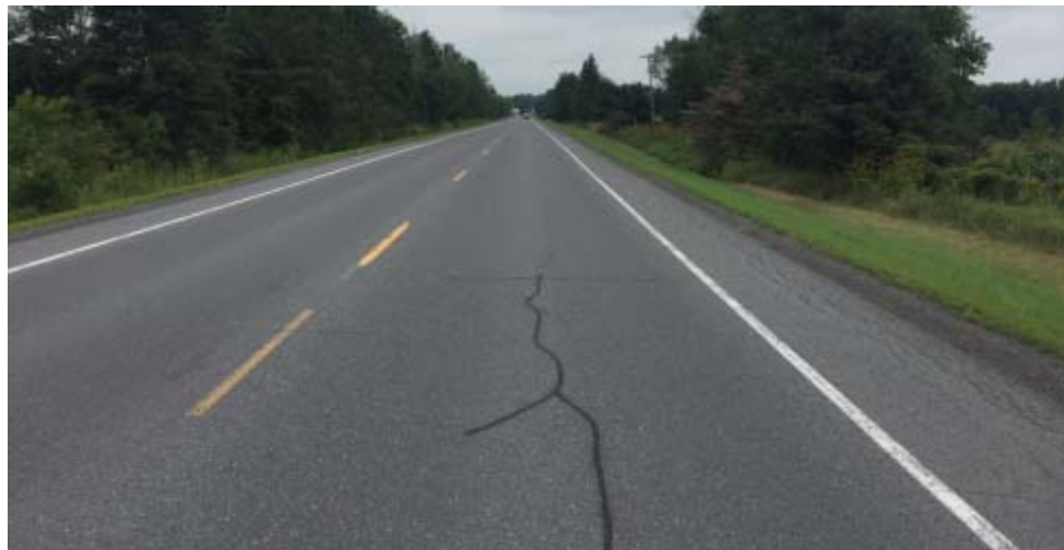
Figure 3-2: County Road 12; Paved surface type (Engtec 2018).
