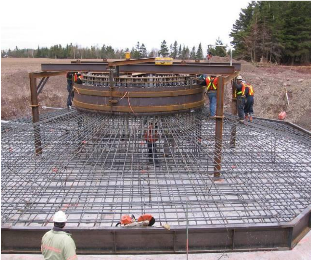
Figure 4-1: Preparation of a typical spread footing foundation
