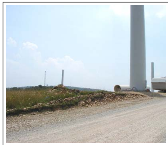
Exhibit 1.5-1 Typical Wind Power Project Gravel Road
