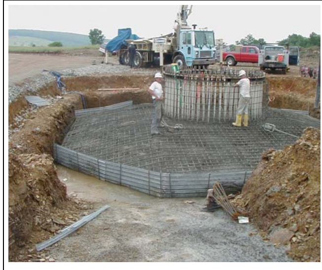
Exhibit 1.5-2 Spread Footing Type Foundation
