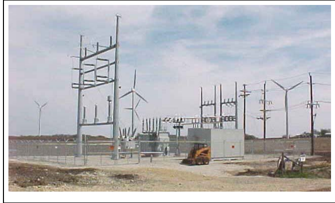
Exhibit 1.5-8 Typical Collection System Portion of Substation Facilities
