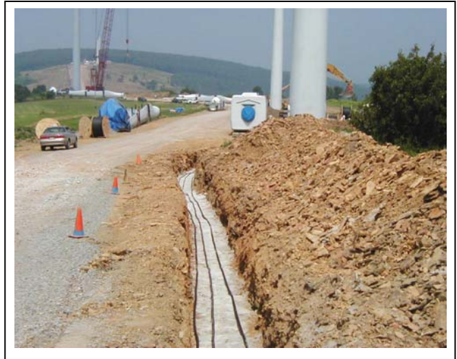
Exhibit 1.5-6 Typical Underground Cable Trench
