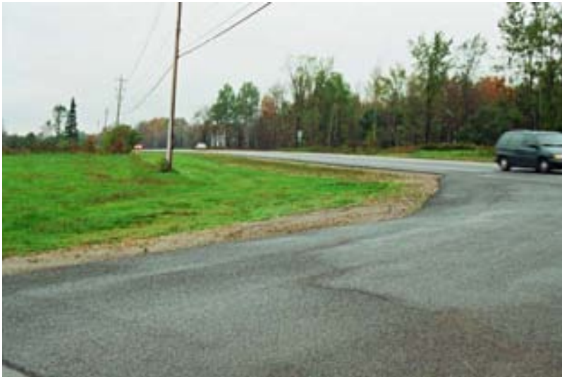
6c. Patnode Rd. (North) at US 11 - SW Corner
