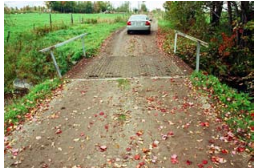
3d. Soucia Rd. – Steel grate bridge
