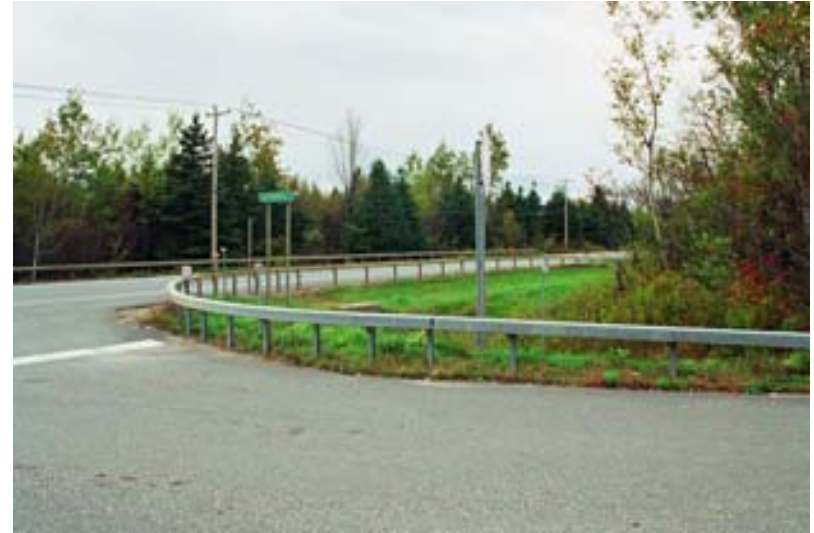
1b. La Francis Rd. at US 11 - NW Corner
