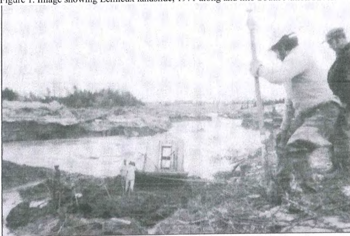
Clearing the channel of leda clay deposits in the South Nation River after the 1971 Lemieux landslide. Courtesy of the SNG.
