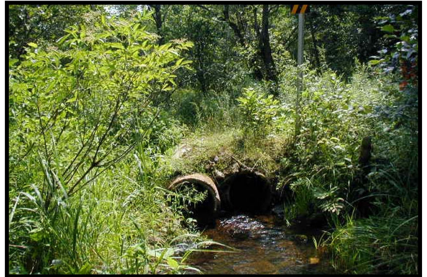
IC969AB-ST facing Southeast
