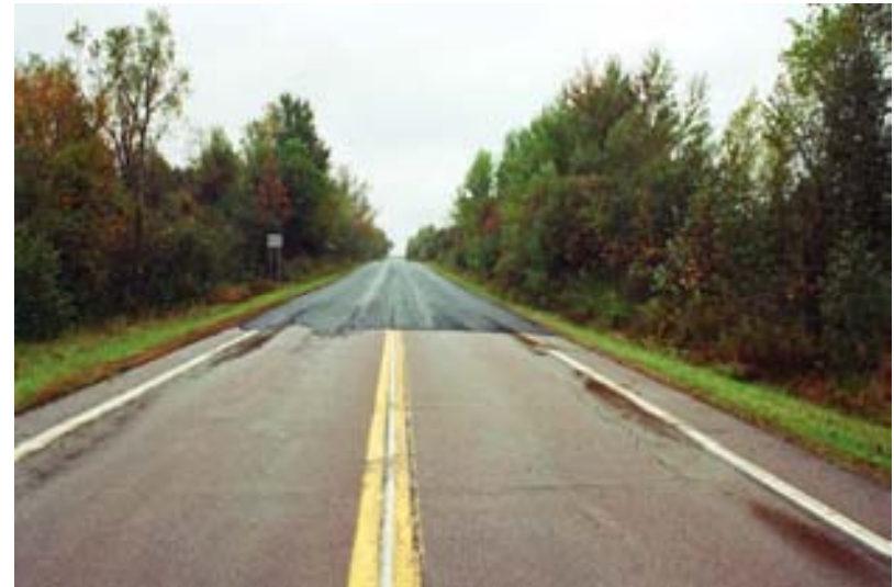
14b. SR 189 – New Overlay - Southbound
