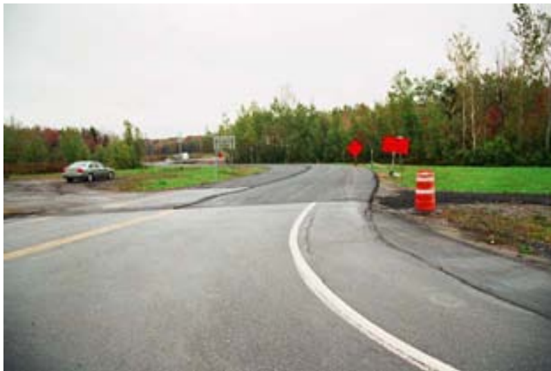
9c. SR 189 – New Overlay - Northbound
