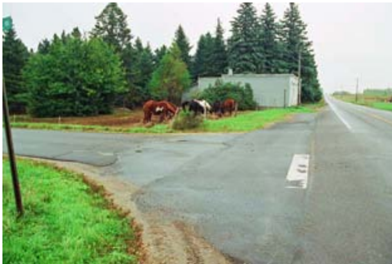
5c. Patnode Rd. (North) at Gagnier Rd. – NE Corner
