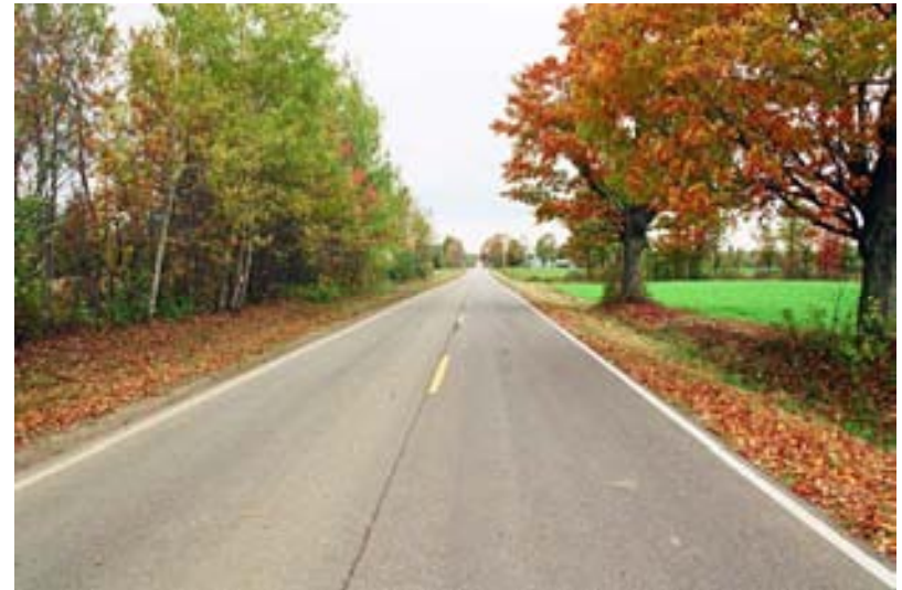
15d. Campbell Rd. - Northbound
