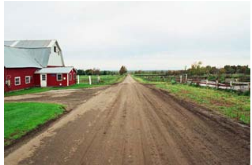
16d. Bohem Rd. at SR 190 - Northbound
