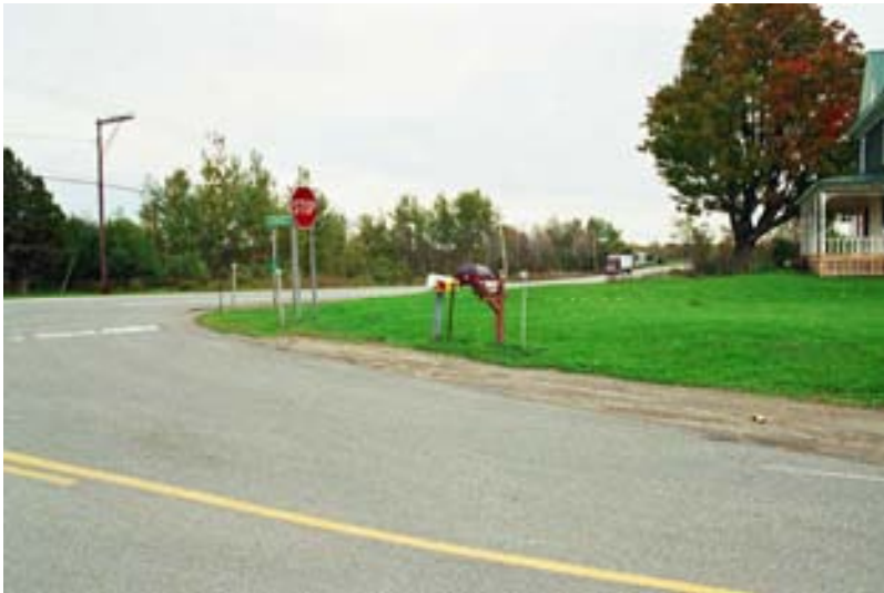
15c. Campbell Rd. at US 11 – SE Corner
