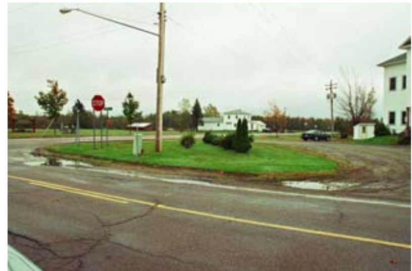
13d. Looby Rd. at SR 189 – SW Corner
