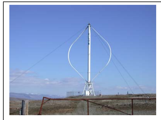
Figure 2. Darrieus Wind Turbine
