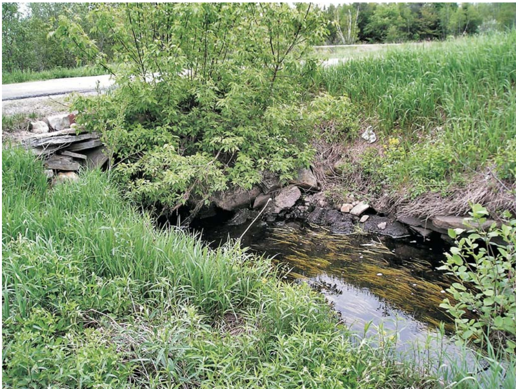
Photograph 14. Channeled and culverted stream under Rogers Road; view to the southeast.
