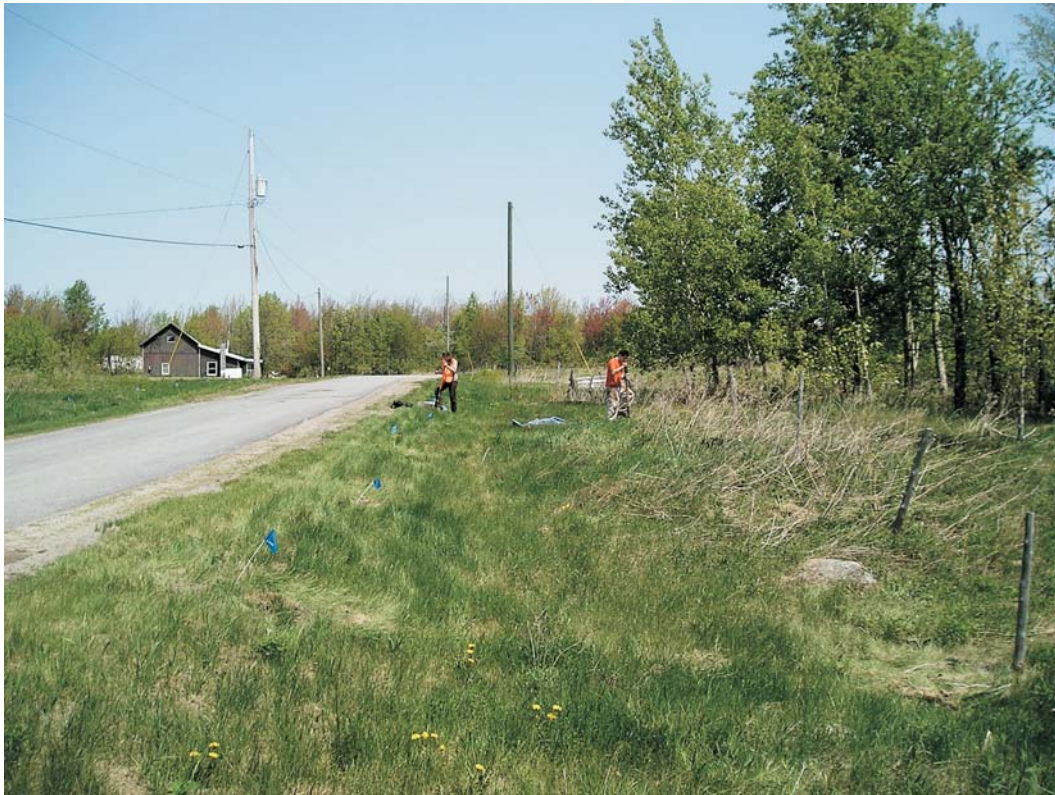
Photograph 13. JMA field personnel excavating shovel tests at Archeological Survey Area C23 – note clump of trees at right indicates location of cellar hole; view to the north.
