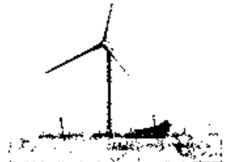
Once complete with 129 turbines— the Maple Ridge Wind Farm in Lewis County will be the largest wind farm east of the Mississippi and will power more than 160,000 New York homes.
