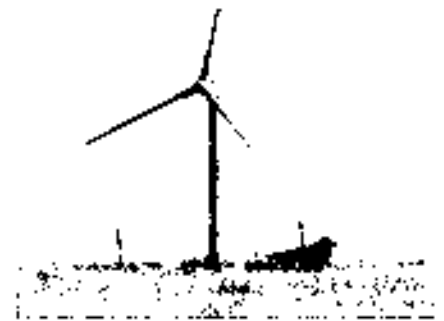
Once complete - with 120 turbines - the Maple Ridge Wind Farm in Lewis County will be the largest wind farm east of the Mississippi and will power more than 100,000 New York homes.
