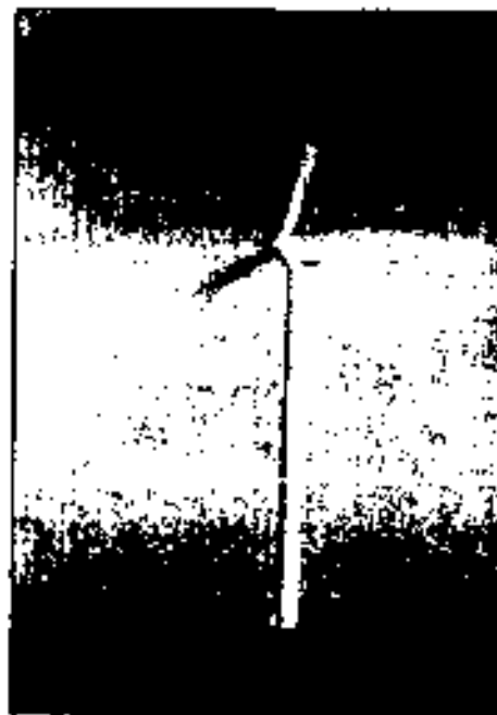
FIGURE 6.1 SOMERSET WIND TOWER
