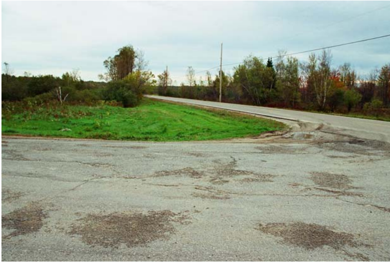
3a. Rogers Rd. at Clinton Mills Rd. – NE Corner
