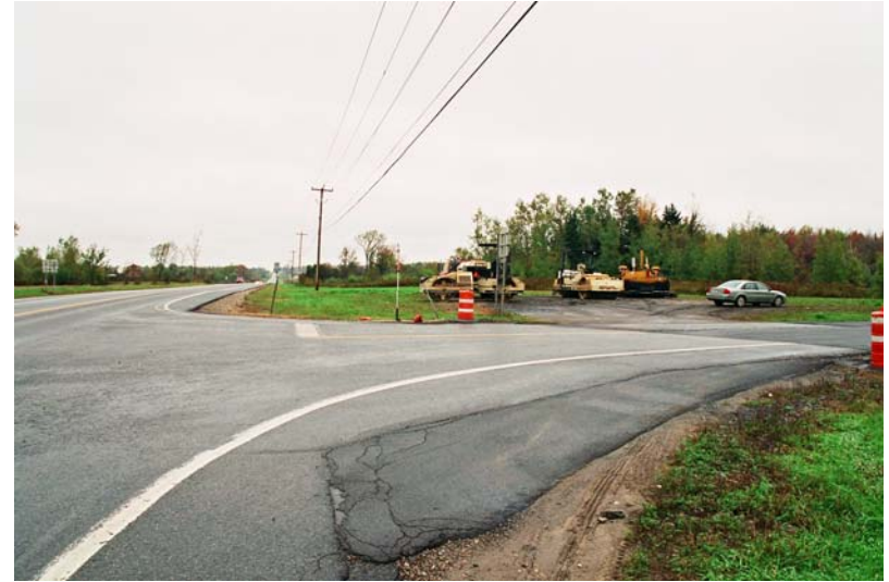
9b. SR 189 at US 11 – NW Corner
