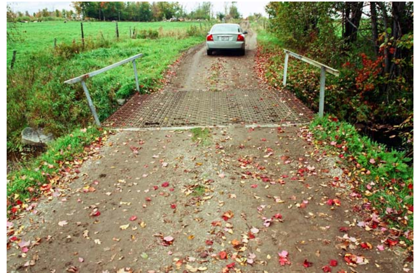
3d. Soucia Rd. – Steel grate bridge
