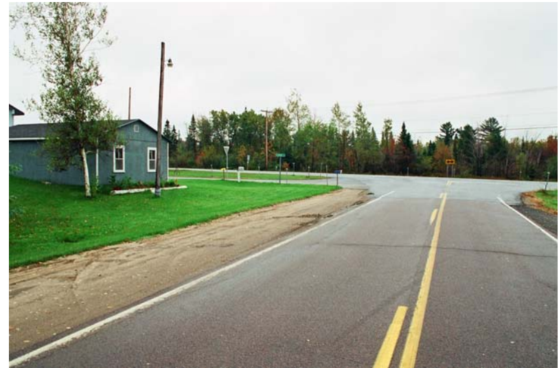
12d. Looby Rd. at US 11 - Southbound
