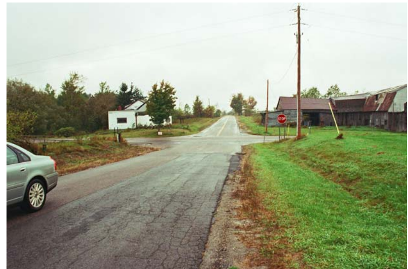
14d. Liberty Pole Rd. at SR 189 - Westbound
