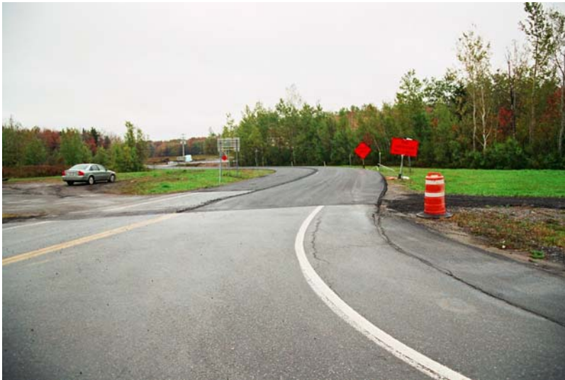
9c. SR 189 – New Overlay - Northbound
