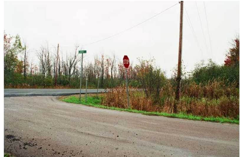
8b. Lagree Rd. at SR 189 – SW Corner
