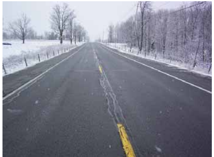
US11 East of Cassidy Rd; Eastbound
