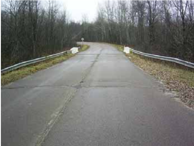
Sweeping 90° Curve; Eastbound
