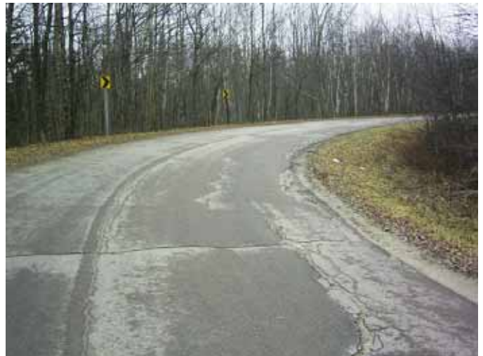
Sharp 90° Curve; Eastbound
