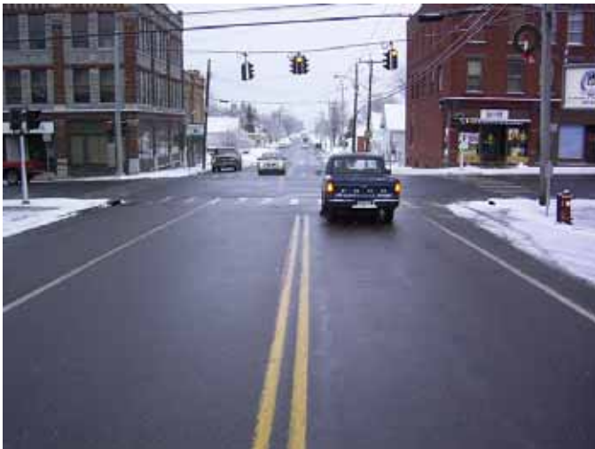
Intersection w/ SR374; Facing North
