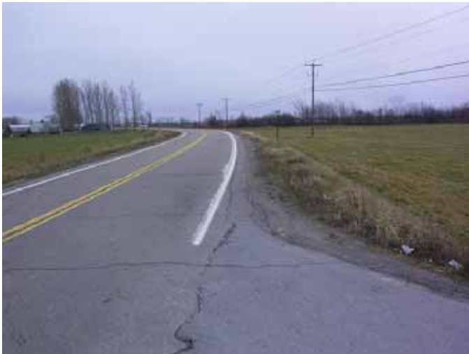
Intersection w/ CR23; Facing East
