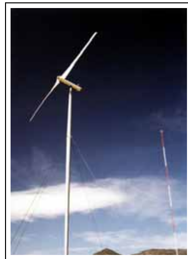
Exhibit 4.5-3 Two-Bladed Downwind Wind Turbine
