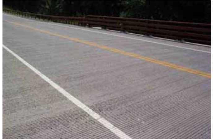
Top of Bridge
