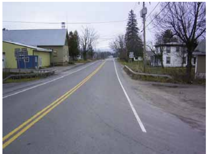
190-24-374 Intersection; Facing South
