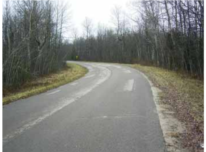
Sweeping 90° Curve; Eastbound
