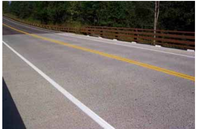
Top of Bridge
