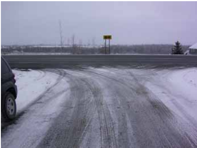
Intersection w/ Cassidy Rd; Facing North
