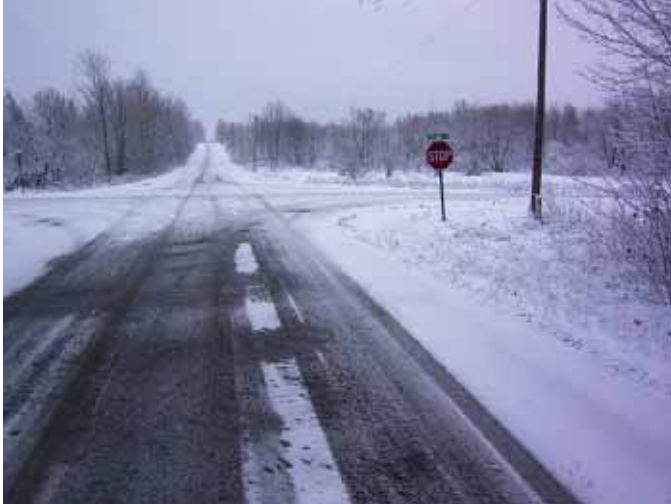
Intersection w/ Sancomb Rd; Facing South
