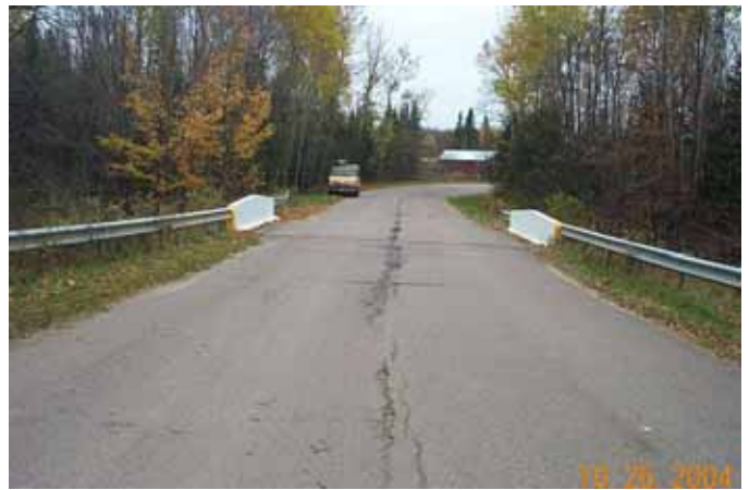
Top of Bridge
