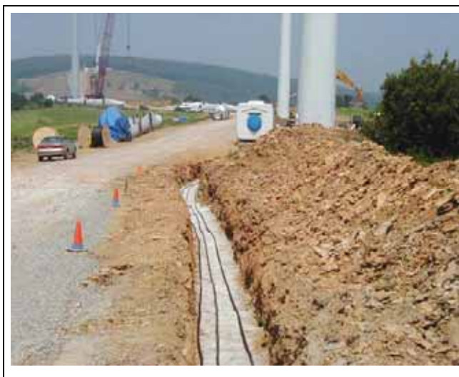
Exhibit 1.5-6 Typical Underground Cable Trench
