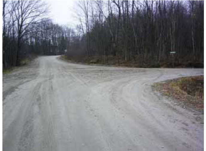
Intersection w/ Ponderosa Rd; Facing South
