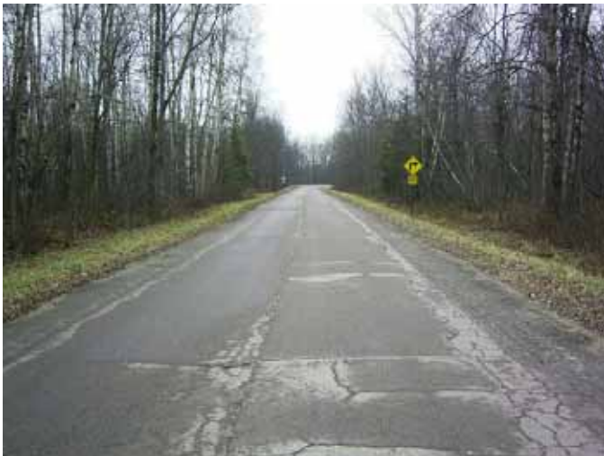
Sharp 90° Curve; Eastbound
