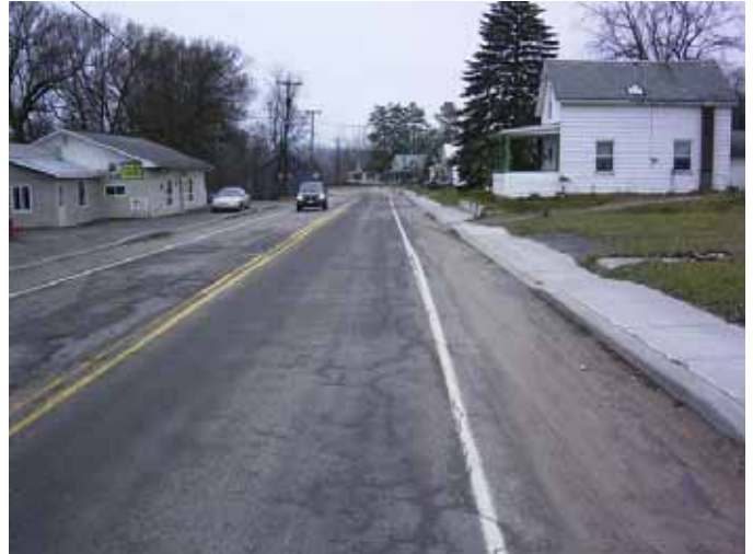
190-24-374 Intersection; Facing West
