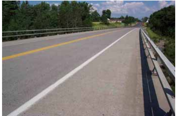
Top of Bridge
