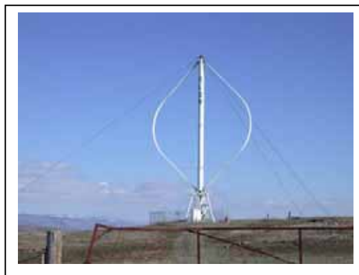
Exhibit 4.5-2 FloWind Vertical Axis (Darrieus Wind Turbine) Located on Thorp Prairie, near Ellensburg, WA
