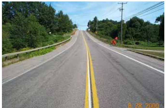
Top of Bridge
