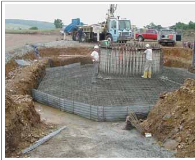
Exhibit 1.5-2 Spread Footing Type Foundation
