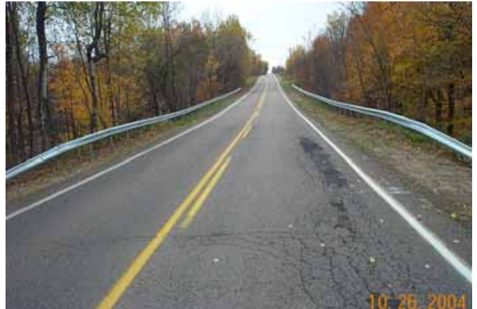
Top of Bridge
