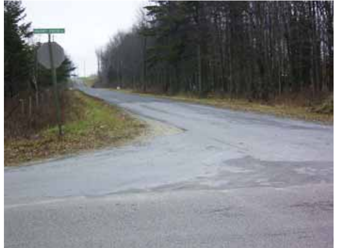
Intersection w/ Legacy Rd; NE Corner
