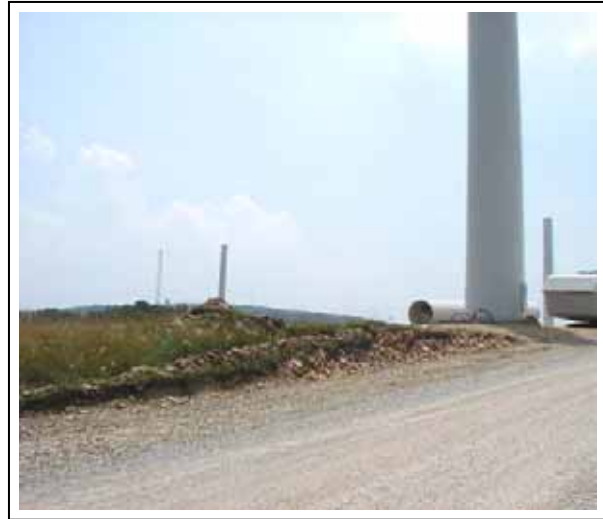
Exhibit 1.5-1 Typical Wind Power Project Gravel Road
